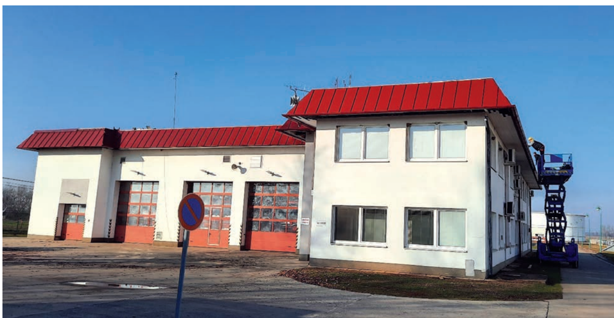
Figure: Roof reconstruction of the ZHÚ facility at PS-1 Budkovce
