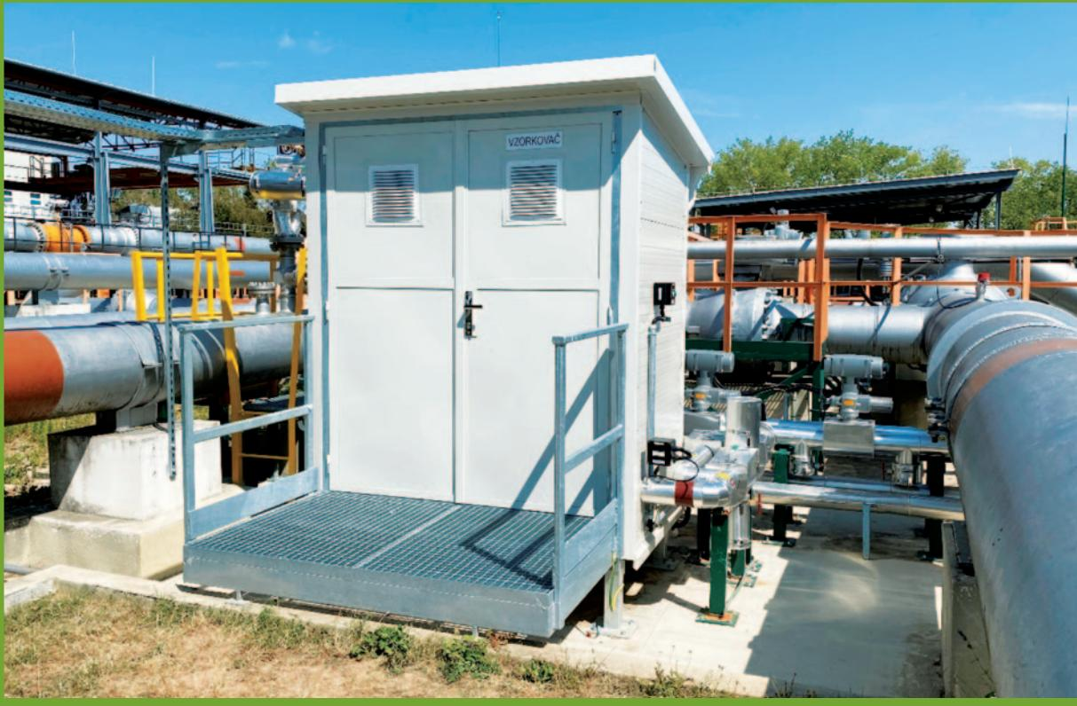
*Photo: Modernised oil sampler at PS5 Bučany*
