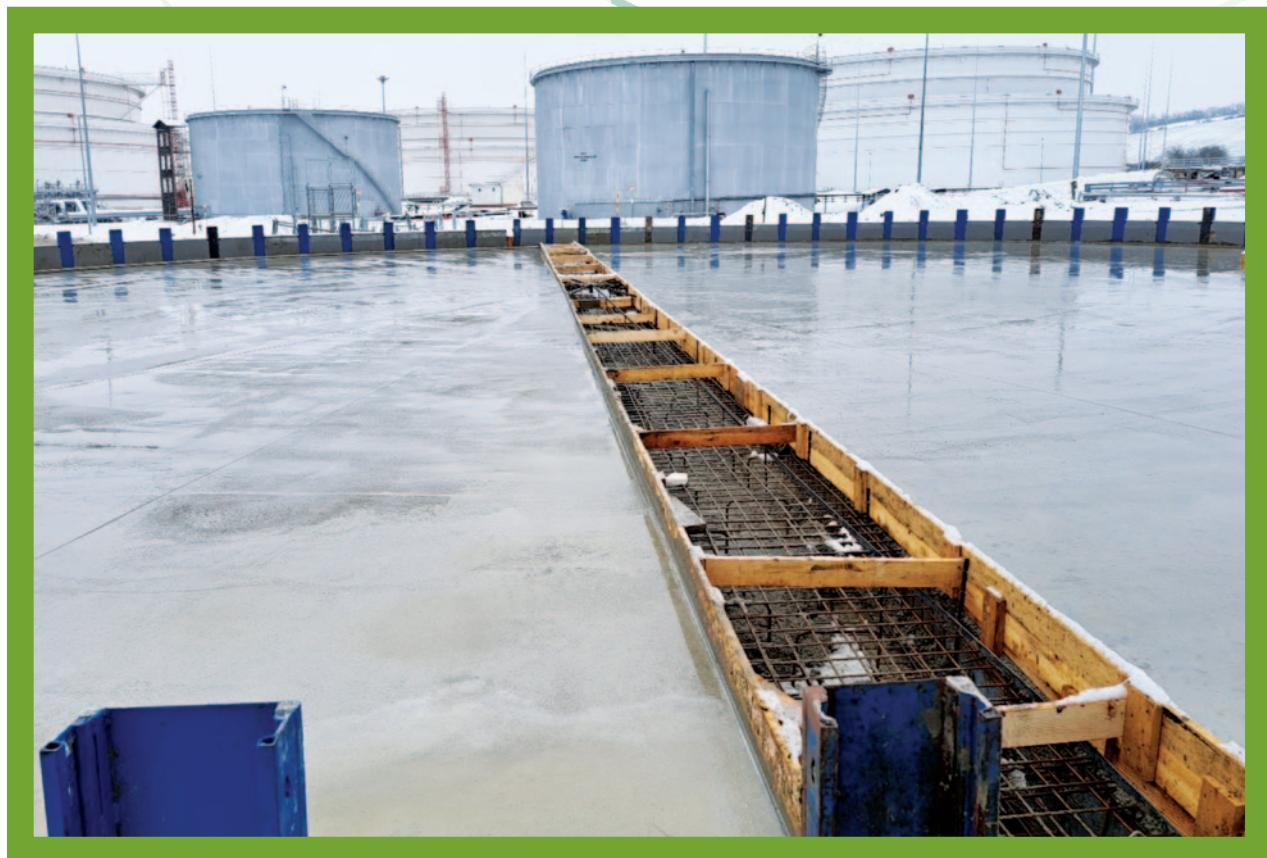
*Photo: Work on the foundation of the new fire water tank; the original fire water and waste water tanks can be seen in the background.*
